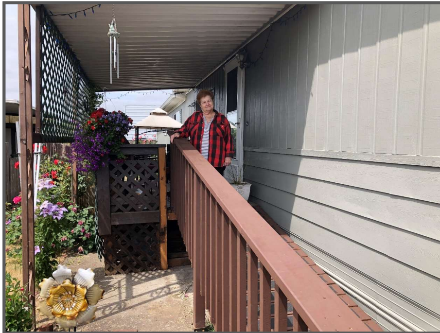
Barbara, new ramp, roof and electrical repairs
