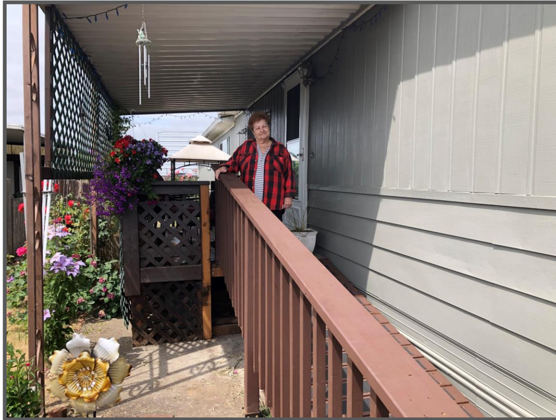
Barbara, new ramp, roof and electrical repairs
